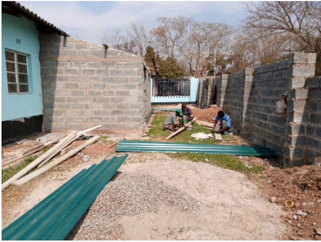
Mounting timber for roofing
