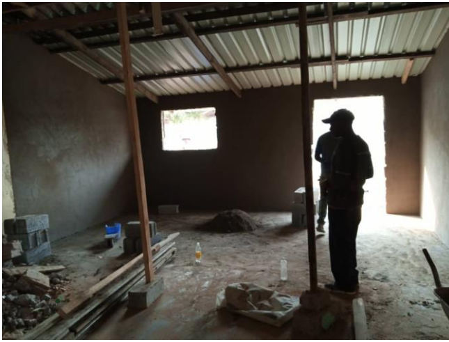
Plastering the expanded labour ward
